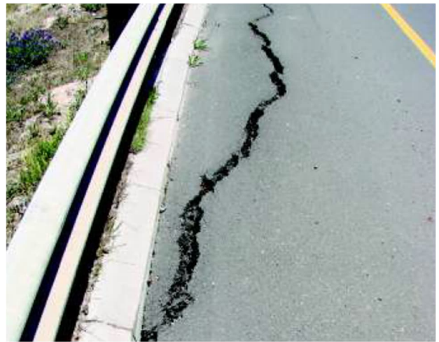
Figure 3.7: Settlement on Fill
