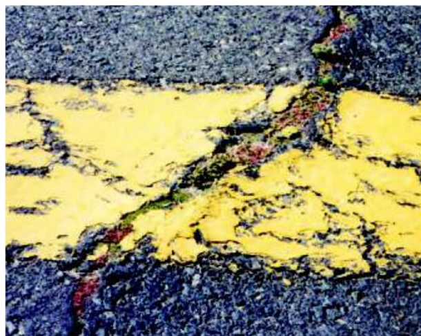
Figure 3.4: Volcano Crack (Active Crack Example)
