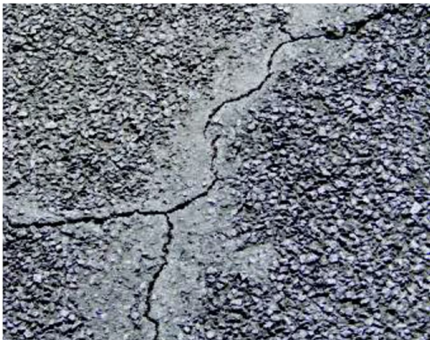
Figure 3.5: Open Surface Crack (Passive Crack Example)
