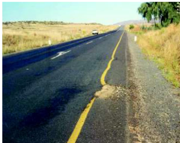
Figure 3.3: Cracking and Rutting (Pavement Failure Example)
