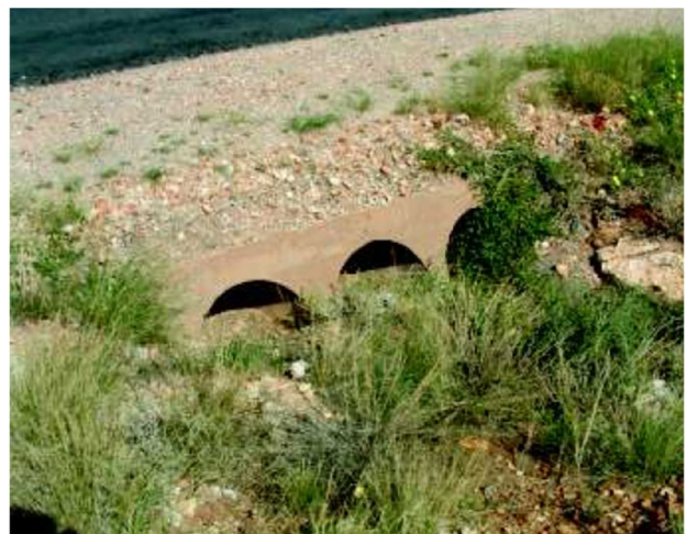
Figure 3.14: Blocked Pipe Culverts
