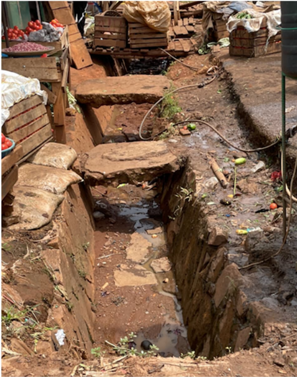
Hazard created by an open drain in Mbale
