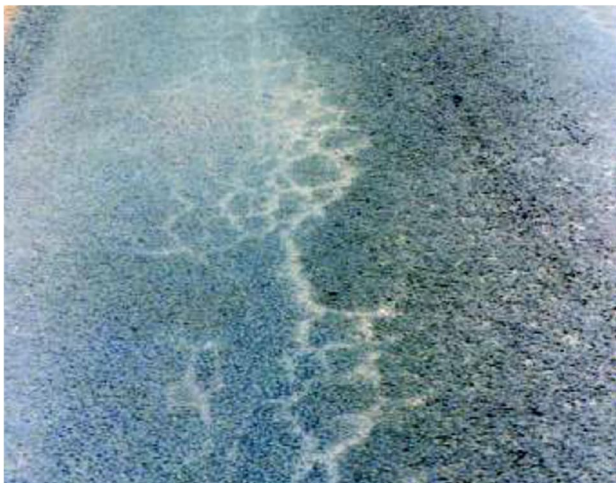
Figure 3.6: Pumping in Wheel Track
