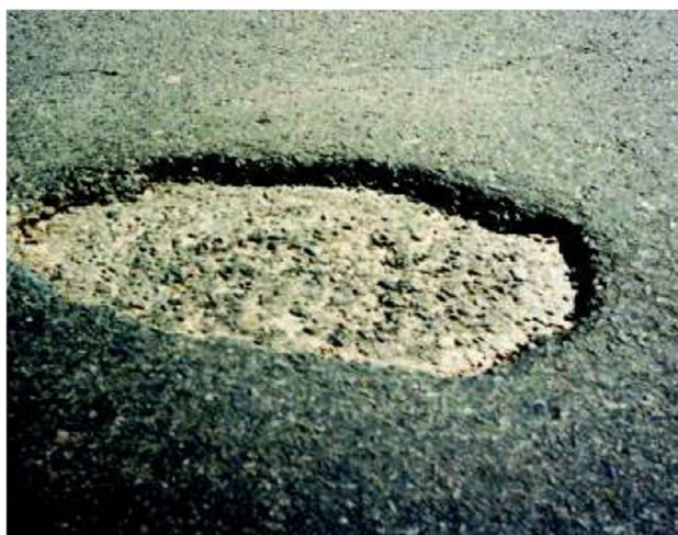
Figure 3.2: Surface Failure Example
