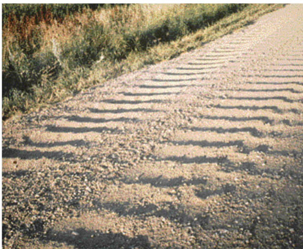
Figure 3.12: Corrugation Source: Gravel Roads Maintenance and Design Manual, SD LTAP
