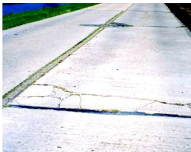
Figure 3.11: Joint Cracks with Weeds
