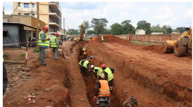
Figure 1.57: Digging Trenches for Water Pipes, Gulu
