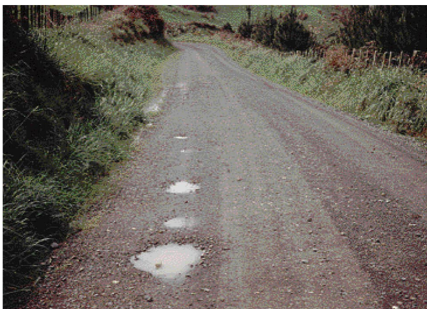
Figure 3.13: Potholes Source: Gravel Roads Maintenance and Design Manual, SD LTAP
